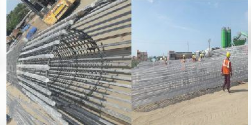
Pamban Bridge -RVNL
